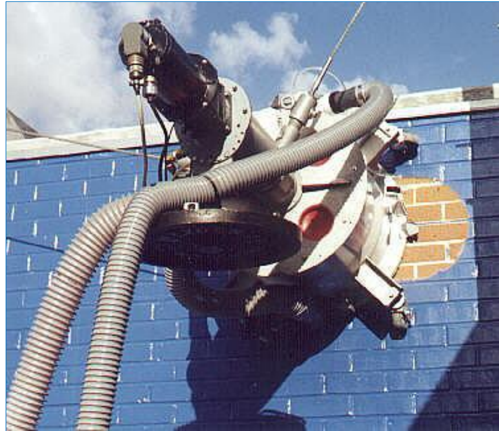
Removal of surface contaminants, including vertical surfaces
